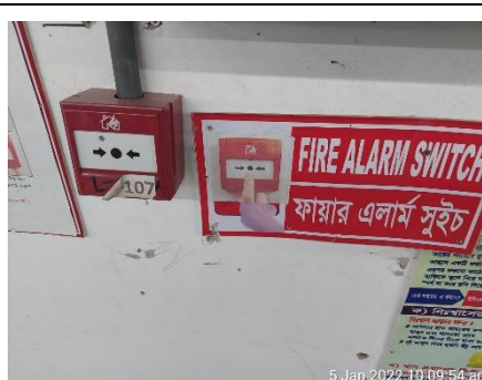
Fire alarm switch
